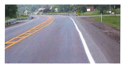
Example of flush divisional island constructed with painting and rumble strip scoring. Alternatively, the island could be constructed of concrete.
